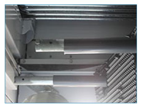
The use of telescopic fill support beams facilates the removal and replacement of the fill sheets.
