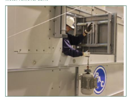
With the motor removal davit, the motor <u>can easily be lowered</u> from or lifted to the motor base without the need for extra heavy material of scaffolding.
