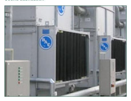
CXVE condensers use **quiet and low kW axial fans**, but to reduce noise even further, you can extend your CXVE condenser with <u>sound attenuation</u>:
