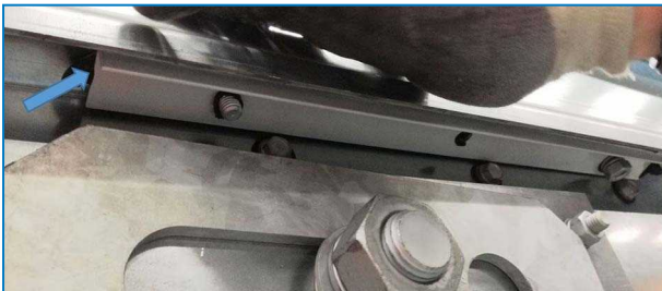
Installed sealing profile
