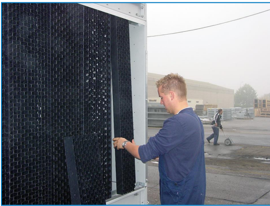
Remove combined inlet shields
