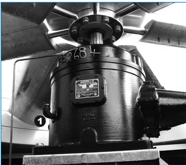
Single reduction gear drive
