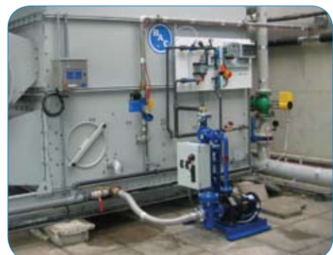
Filtration installation
